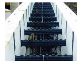
Vertical & Horizontal Clips in place close to corner
