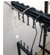
Vertical Clips in Place
