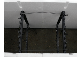
Horizontal Clips in Place
